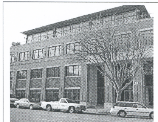
Figure 7. Fenestration and vertical modulation techniques help to reduce the architectural scale of this office building
