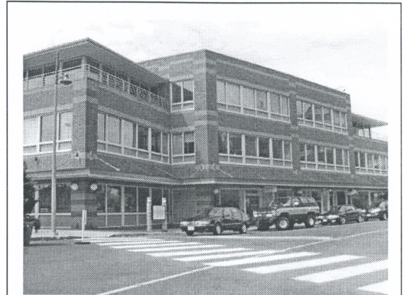
Figure 9. Use of building modulation, window patterns, brick, balconies and awnings help lend this building a human scale.
