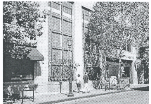
Figure 6. This parking garage includes street front retail space and landscaped trellises to mitigate visual impacts
